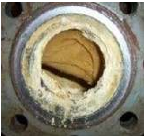
Pipe Interior Before Treatment
